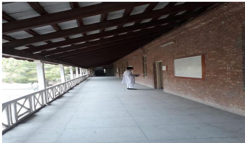
Fig. 5. Roof With Wooden Materials
