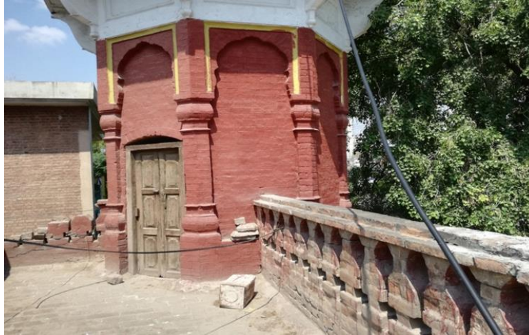
Fig. 9. Irregular Story Heights of the Building
