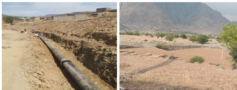
Figure 3: Water supply line at Gandao town Figure 4: Agricultural Land of the study area
